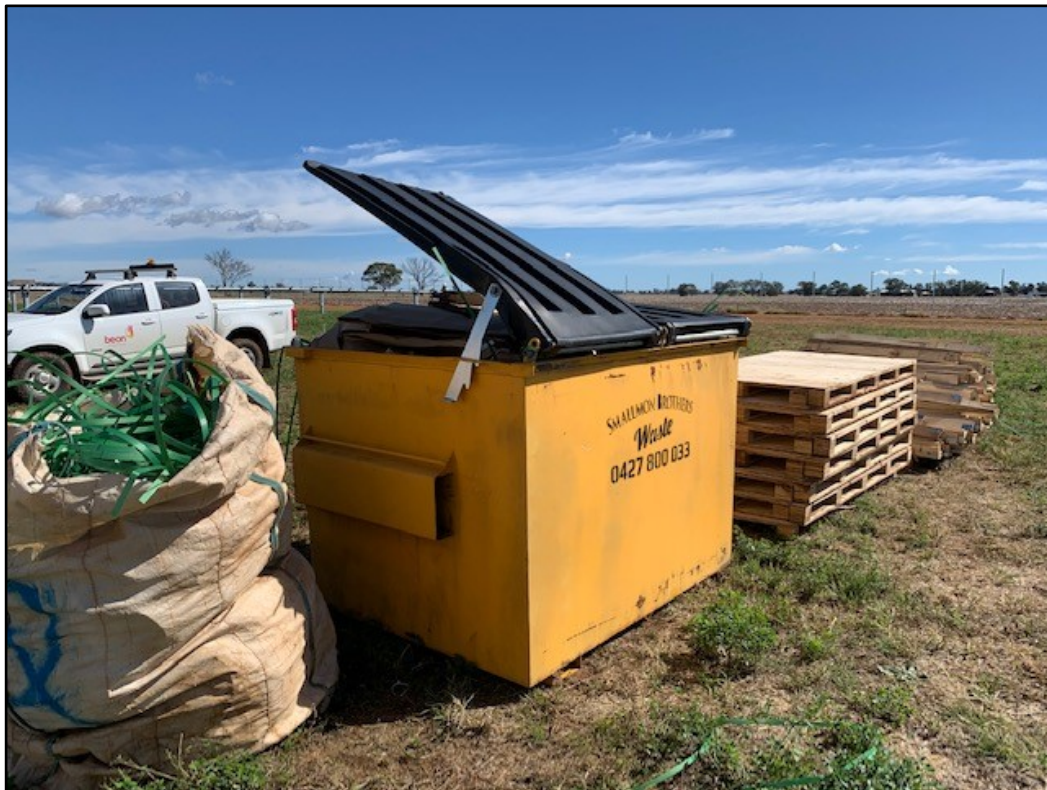
Plate 7: View of segregated construction waste and re-use materials prior to off-site transport for recycling or disposal. General housekeeping was noted to be of a very high standard across the project site.
