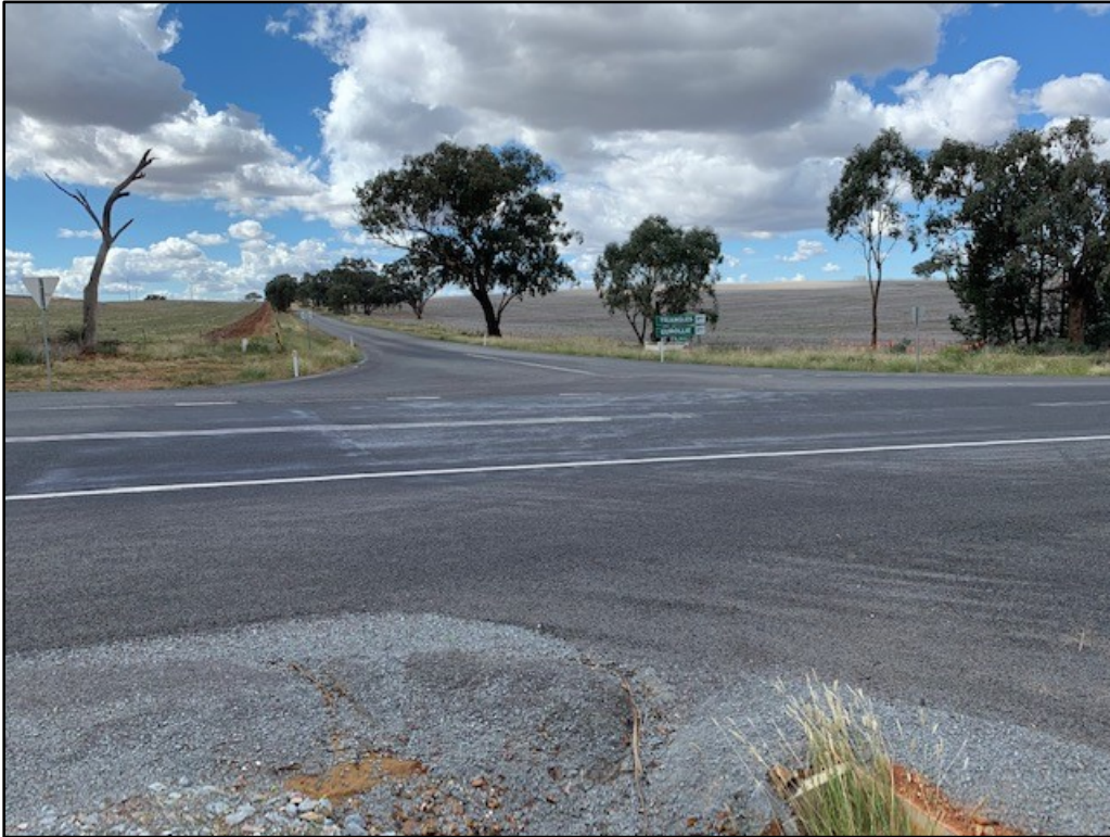
Plate 1: View of the upgraded Eurolee Road, looking east from the intersection of the Goldfields Way. The distance of new asphalt seal on Eurolee Road was measured during the audit to be approximately 400m from the intersection.
