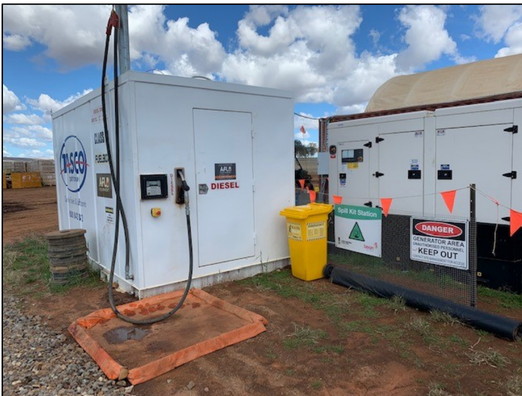
Plate 6: View of the site fuelling area at the time of the auditor's site visit on 26/03/21. An appropriately stocked spill kit was noted to be present along with signage, bunded storage and a portable spill containment bund.
