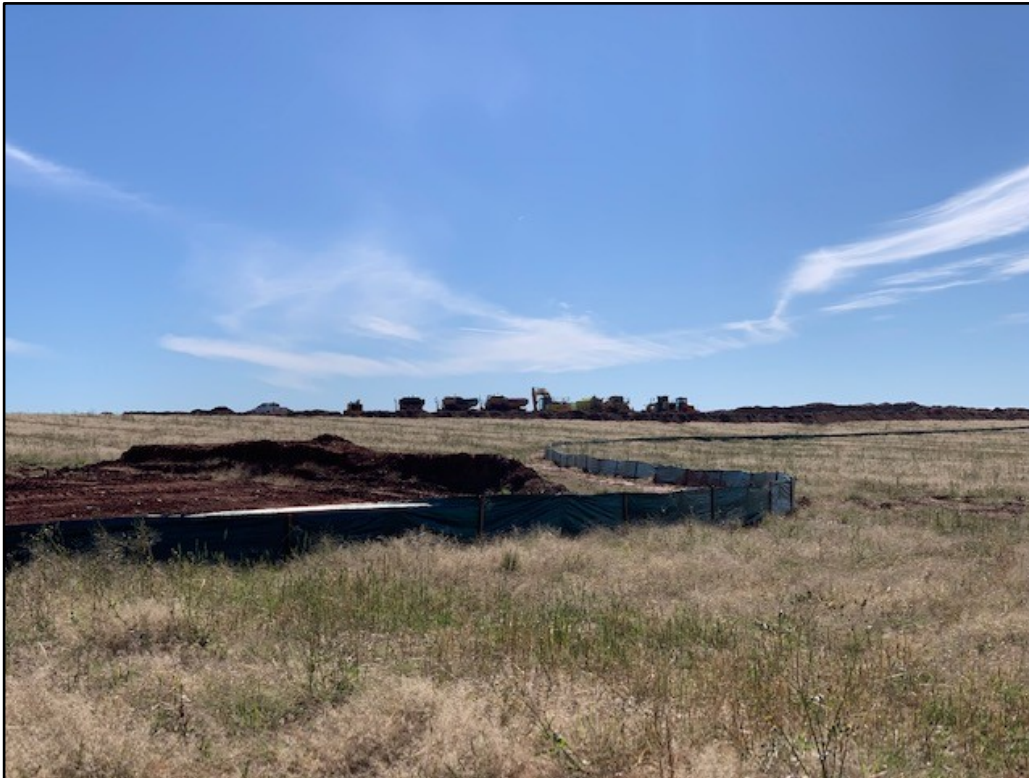
Plate 3: View of the sediment fencing and water quality basin installed on the southwest portion of the site as part of the Project erosion and sedimentation control measures documented within the Soil and Water Management Plan. No evidence of significant sedimentation and/or erosion was noted during the Auditor's site visit of 26/03/21.
